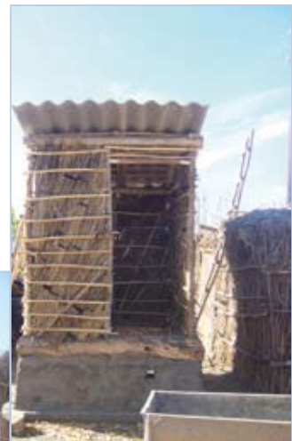
EcoSan toilet constructed with reed walls, which are then covered with daub, a cheaper building material than bricks.
