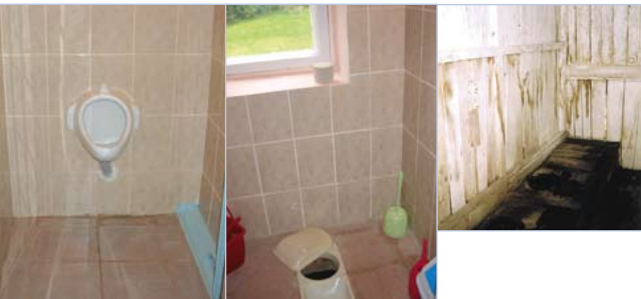
Bad-smelling pit latrines (3) were replaced by a dry urine diverting indoor toilet (2) and urinals (1) (source WECF).
