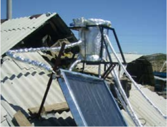
A solar collector provides warm water for laundry and shower
